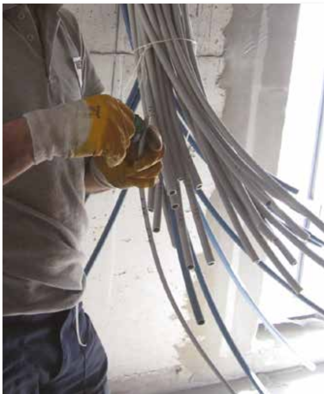
An operator stripping cables during installation.
